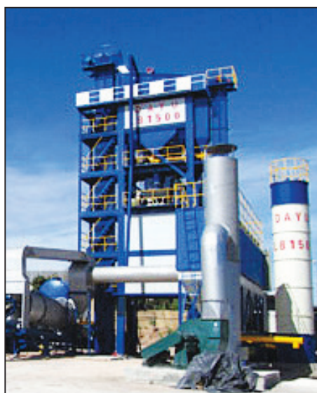
The plaintiffs sought to challenge the issuance of a special permit for an asphalt plant near the Chelmsford line.
